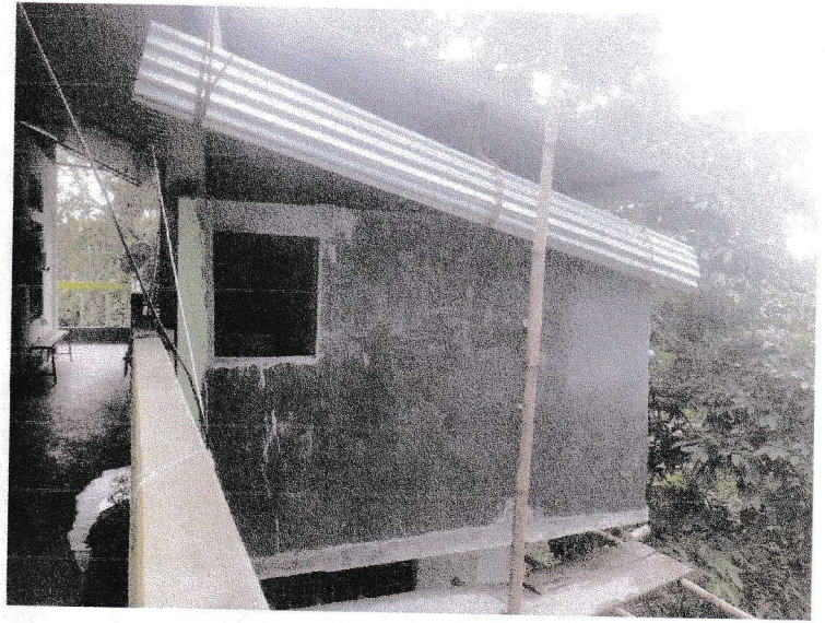
Rain Water Harvesting
